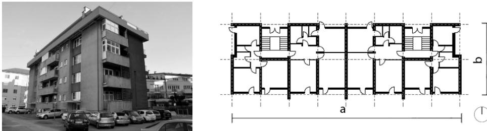
Figure 2. Existing case study building – EB B (left) and its floorplan (right)
